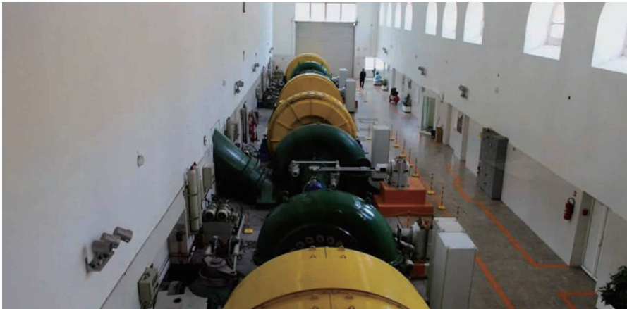
The Miljacka powerhouse contained four turbine-generator units when at full capacity
