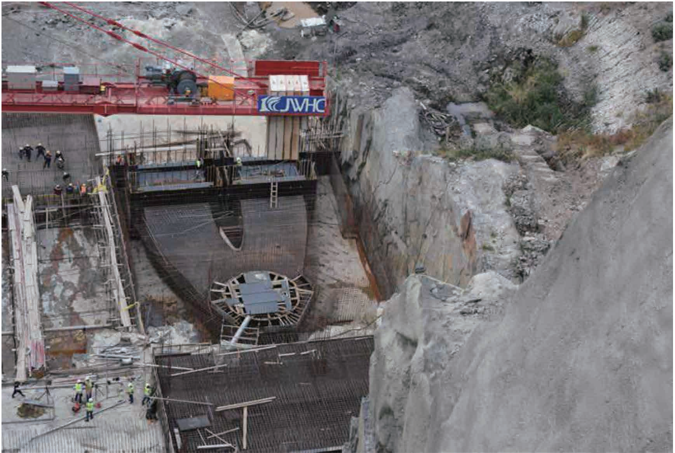
Formwork and Preparations to Cast Concrete for Unit 3 Draft Tube, Rusumo Falls Hydroelectric Project, Nov 2019
