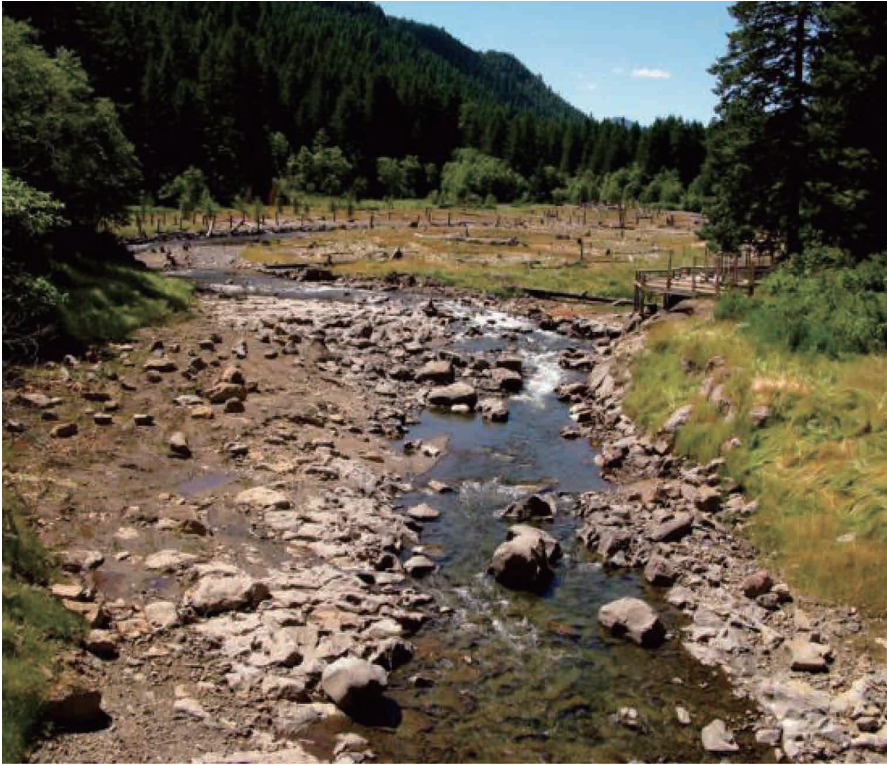
A reconstructed section of Trout Creek in Washington runs through the site of a former reservoir in 2010, a year after Hemlock Dam was removed Inter-Fluve/USDA Forest Service, Gifford Pinchot National Forest
