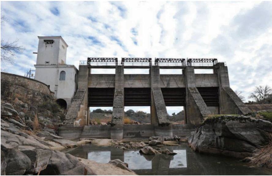
The Yecla de Yeltes Dam in Spain is being demolished in the largest project of its kind ever in Europe. Credit: Dam Removal Europe
