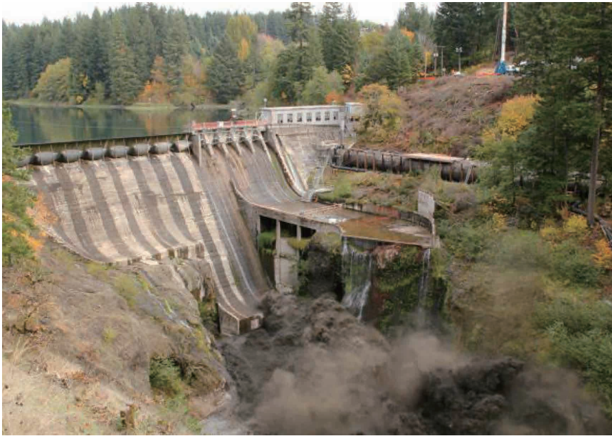
In 2011, the Condit Dam was destroyed by breaching the base of the structure
