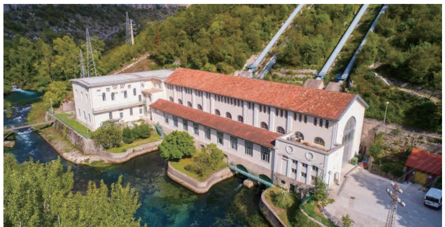
Exterior of the powerhouse for the Miljacka hydropower plant
