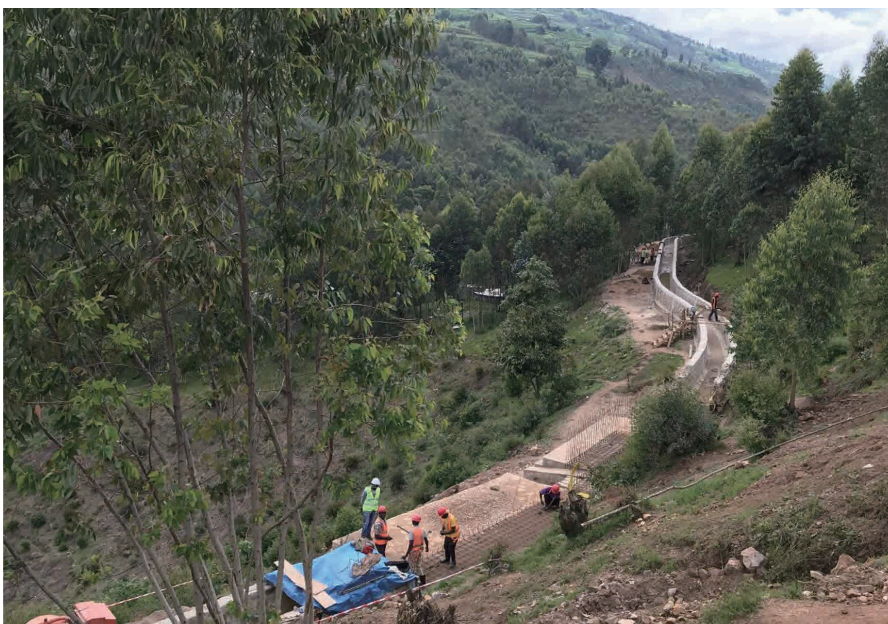
Kavumu SHPP (0.334 MW) Channel under Construction, Nov 2019 (Photo by ZHAO Jianda)
