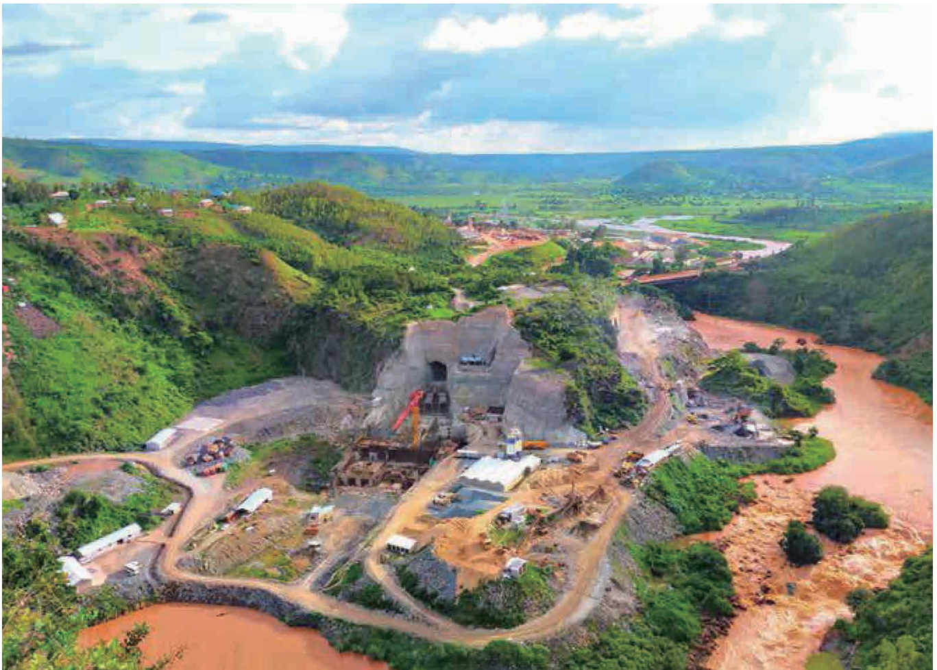
Powerhouse Construction Works, Rusumo Falls Hydroelectric Project, Nov 2019
