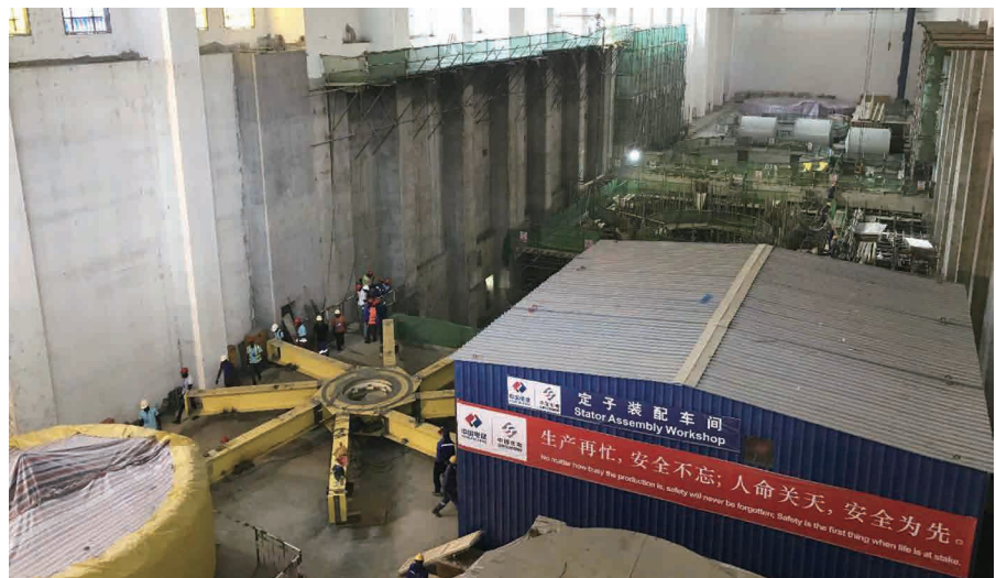
The Powerhouse under Construction, Nov 2019(Photo by ZHAO Jianda)
