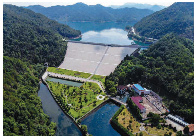
Figure 4. Hengjin First Cascade in Zhejiang Province (9,750 kW)
