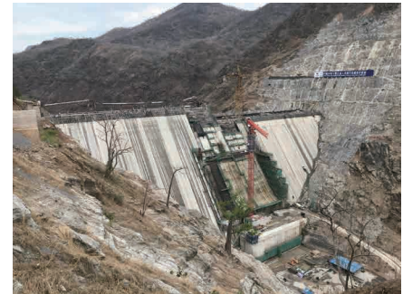
The 139.0m-high RCC Dam under Construction, Nov 2019 (Photo by ZHAO Jianda)
