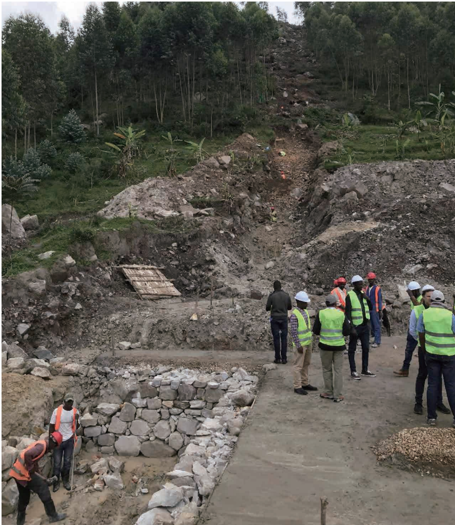
Kavumu SHPP (0.334 MW) Powerhouse and Penstock under Construction, Nov 2019 (Photo by ZHAO Jianda)
