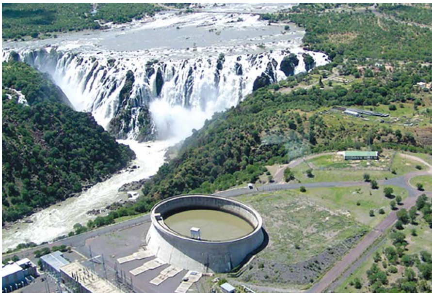
General View of Namibia Ruacana Hydro Project
