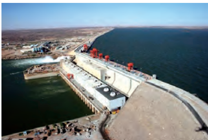
The Merowe hydropower dam of Sudan
