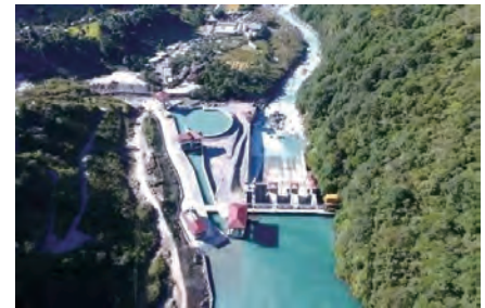
Marshyangdi Hydropower Plant (A)
