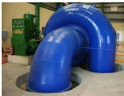
Moa HEPP in Cuba (2×1MW)
