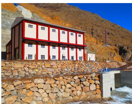
Ozluce HEPP in Turkey (2x18.9MW)
