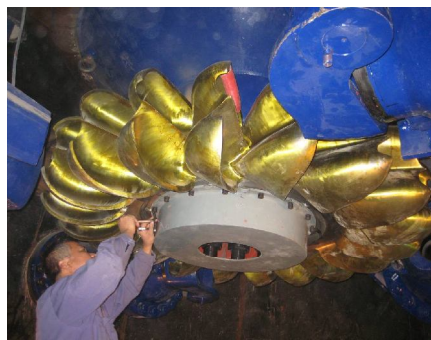
Runner installation for four-jet Pelton turbine
