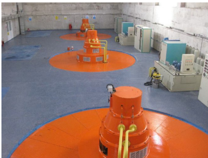
Kale HEPP in Turkey (3×13MW)
