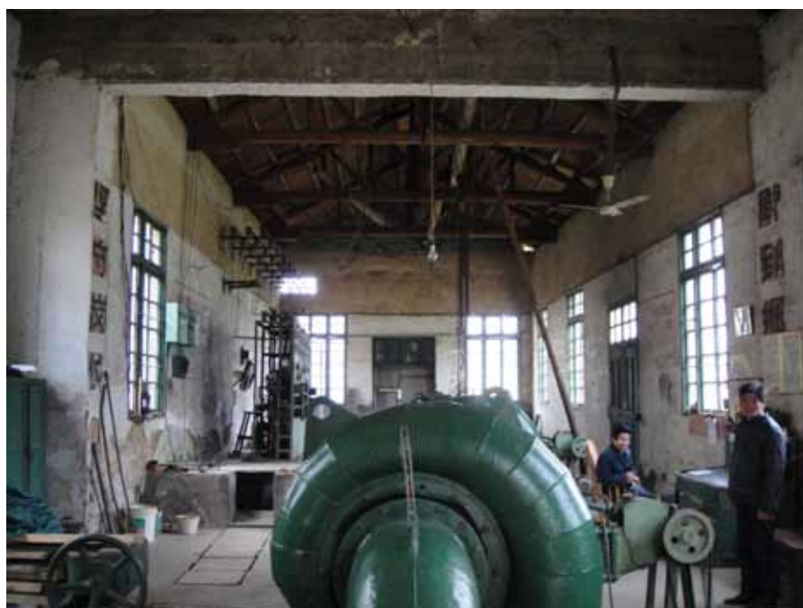
Fig 1: An old SHP powerhouse and its generation equipment need to rehabilitate
