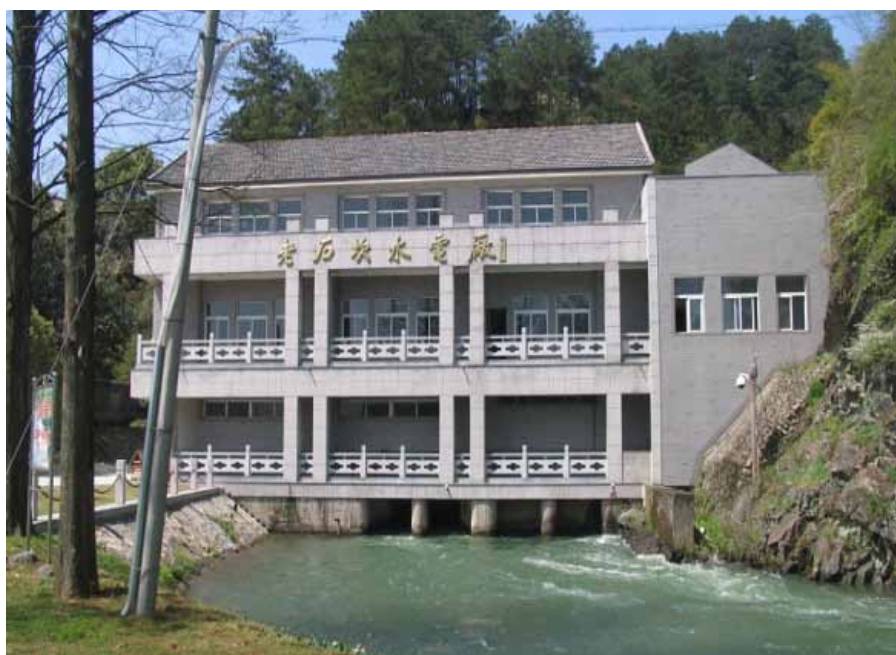
Fig 3: Laoshikan SHP station, located in Anji county, Zhejiang province, firstly commissioned in 1968 with total installed capacity 1,860 kW (1,360 kW+500 kW) and annual generation in design 5 \times 10^6 kWh. After two technical renovation in 1986 and 2005, presently its installed capacity reaches to 3,500 kW (2,500 kW+1,000 kW) and annual generation in design is 13 \times 10^6 kWh. Safety, reliability and generation efficiency are well improved after application of computer monitor and control technology.
