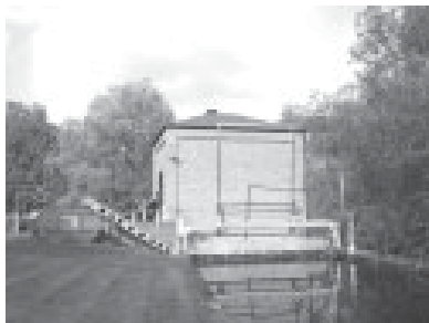
Fig6-1. Nykvarn Micro Hydro Power in Linköping, Sweden(325kW), an excellent example of environmental friendly SHP. A trash-rack cleaner is individually designed by the plant self
