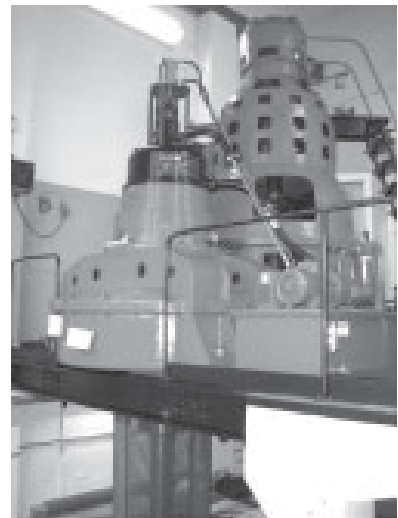
Fig 6-4. A 325 kW turbine manufactured in 1942 still kept in operation
