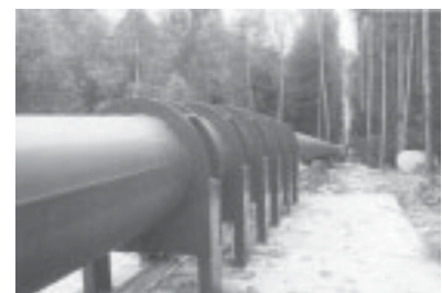
Fig 4-1. An uncovered anchoring block at penstock without expansion joints
