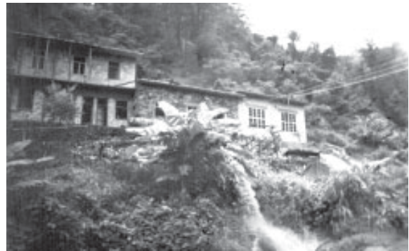
Fig 4-3. A powerhouse coated with local stone
