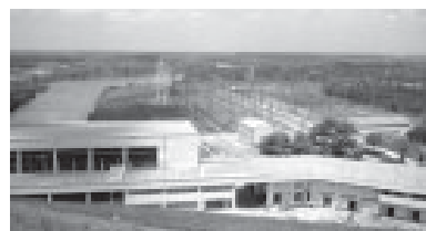
General view of powerhouse and 220kV switchyard (on the upstream side)
