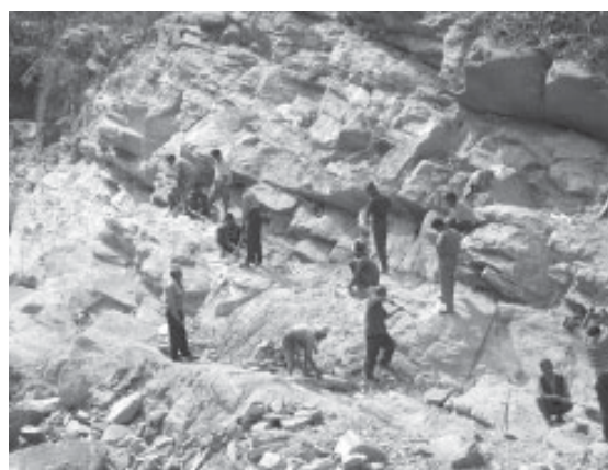
Fig. 3: Chiseling of Hard rock at Piluwakhola Project
