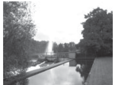
Fig 6-3. Intake of Nykvarn MHP
