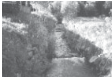
Fig 4-2. An excellent example of fish friendly nature-like fish way with step and pool morphology [12]
