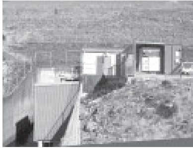
Fig.6-6 Parangana Dam SHP plant(1×750kW), a containerized SHP station in Tasmania State, Australia
