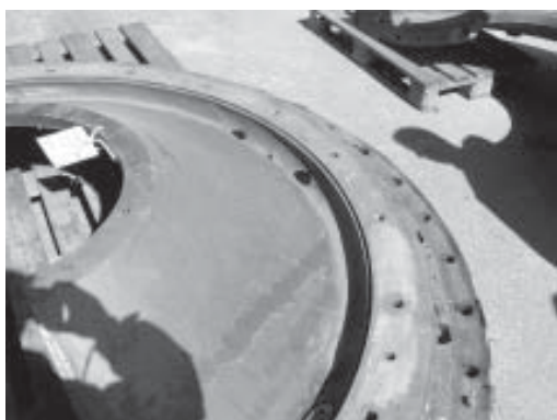
Figure 3: Damage in headcover of old Francis turbines
