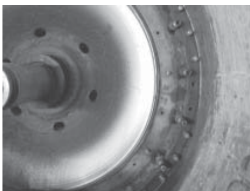
Figure 4: Sediment-laden water passes through the gap (3 mm) between runner and turbine casing
