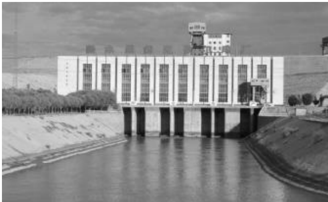
Kezier water reservoir built at the end of 1980's is located on the crossing site of Muzati river and Kezier river. It has integrated multiple functions, with main function on irrigation, flood control, as well as power generation. The installed capacity of this hydropower plant is 26,000kW. The total investment is 385 million Yuan RMB.
