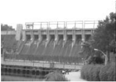
Visit to Xinanjiang Hydropower Station, the 1 st one designed and constructed by Chinese
