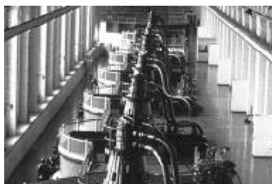
Safe Harbor dam generators, Pennsylvania (Safe Harbor Water Power Corp).
