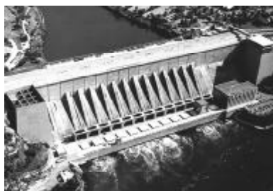
Robert Moses dam, New York (New York Power Authority).
