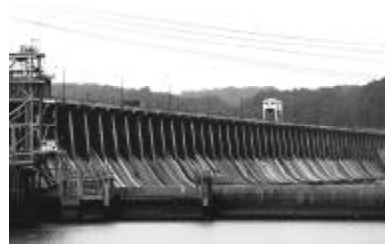
Conowingo dam, Pennsylvania (Susquehanna Electric Company).
