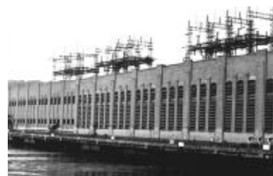
Safe Harbor dam, Pennsylvania (Safe Harbor Water Power Corp)
