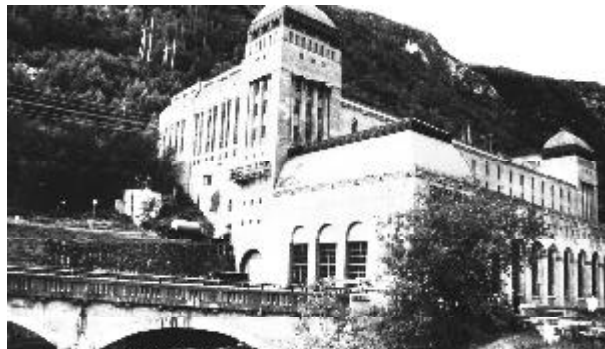
Fig. 8. Saaheim power station (108 MW in 1916, 189 MW in 2002).
