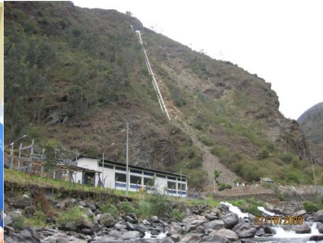
Sandia hydropower plant is situated in far southeastern Peru in Puno province, 15km to Sandia downtown. It is a small run-of-the-river type with an installed capacity of 1200kW and a water head of 220m, and it is also the first Pelton project for Hangzhou Yatai awarded in overseas market.
