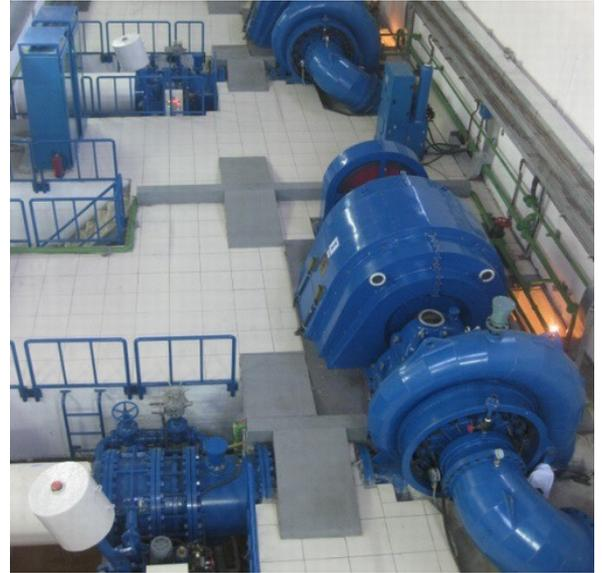
Invested by H.G.M. Enerji İnş. Nak. Gıda Gb. Yem San. ve Tic. Ltd. Őti., Keklicek hydropower project is at suburban area of Malatya in the southeast of Turkey. The water head of the power plant is 166m and it consists of 2 horizontal Francis turbine-generator units with total installed capacity  $2 \times 4337 \text{kW}$ . Hangzhou Yatai supplies the electro-mechanical equipment and achieves the acceptance and commercial commissioning in July 2009.
